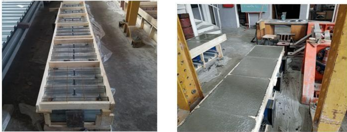
Figure3. Casting of concrete
